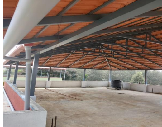
Office New Roof
