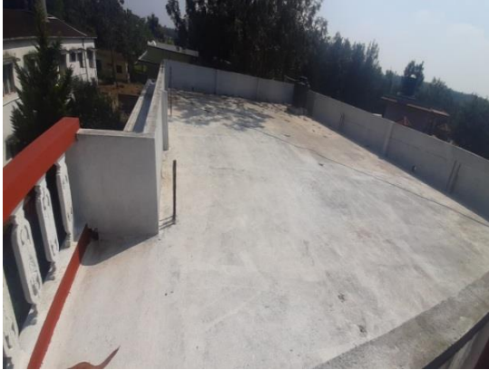
Office Old Roof
