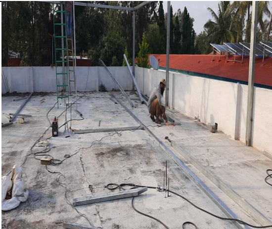
Staff QTR Roof before
