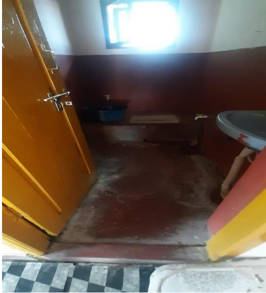
Staff QTR Toilet Before
