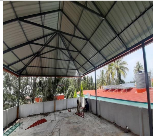
Staff QTR Roof after
