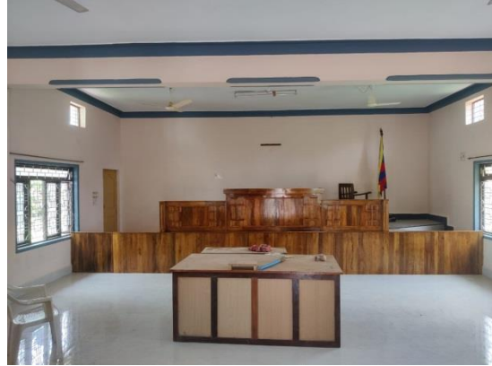
After flooring and Wood partition
