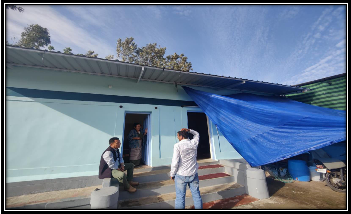
House renovation TDL Camp 03 house no 04 (Mrs. Choekyi ) amounting rupees 364,400.00
