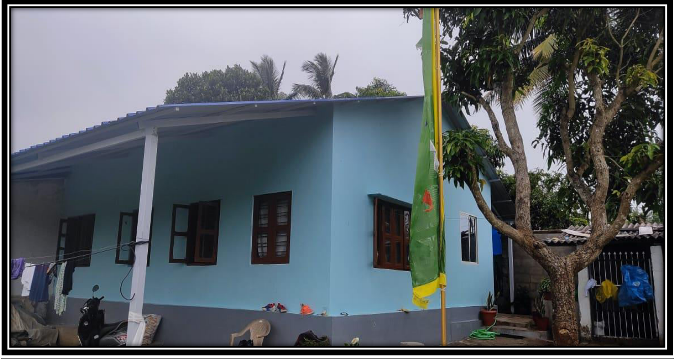
House renovation TDL Camp 02 house no 11 (Mrs. Tenzin Youdon) amounting rupees 515,870.00
