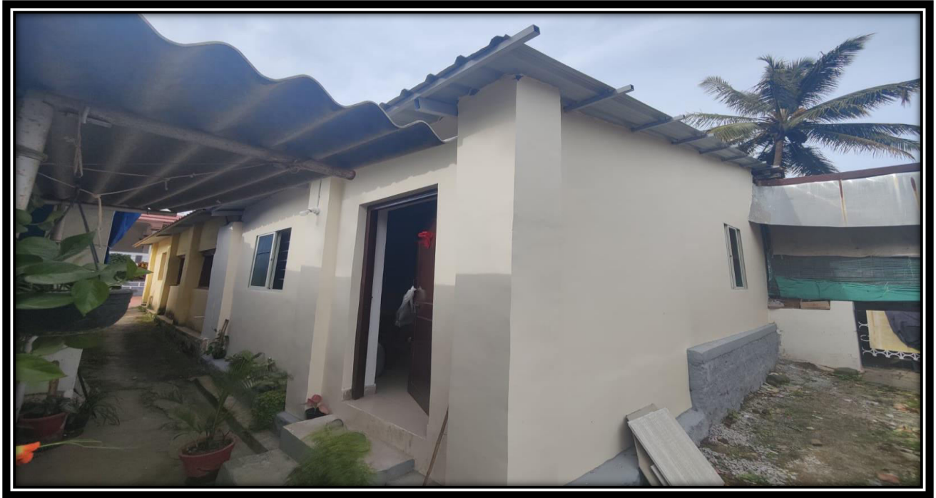
House renovation TDL Camp 08 house no 15 (Mr. Lhakpa Kilu) amounting rupees 340,000.00
