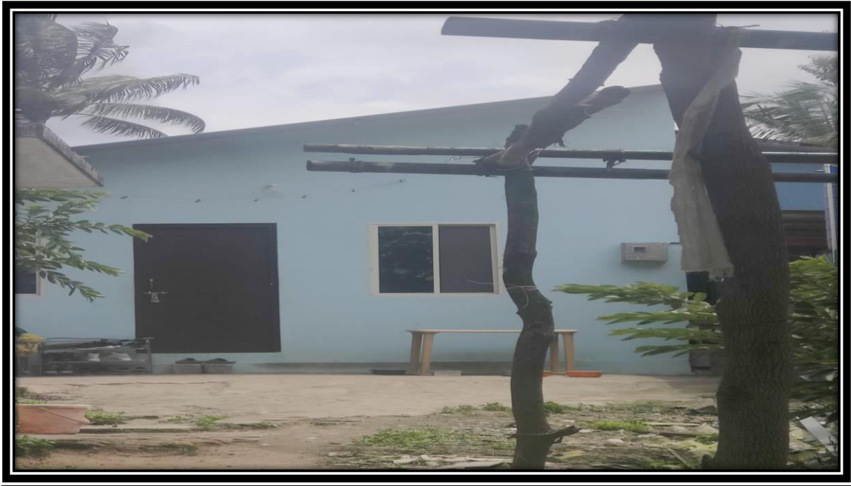
House renovation TDL Camp 02 house no 19B (Mrs. Tashi Yangzom) amounting rupees 445,210.00
