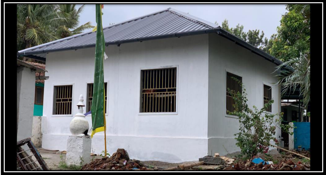
Roofing Installation TDL Camp 10 house no 17 (Mrs. Palzom) amounting rupees 120,000.00
