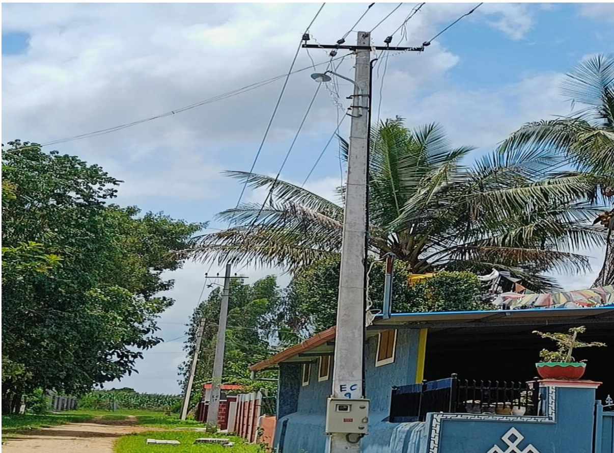
Installation of electricity meter with time at electric pole.
