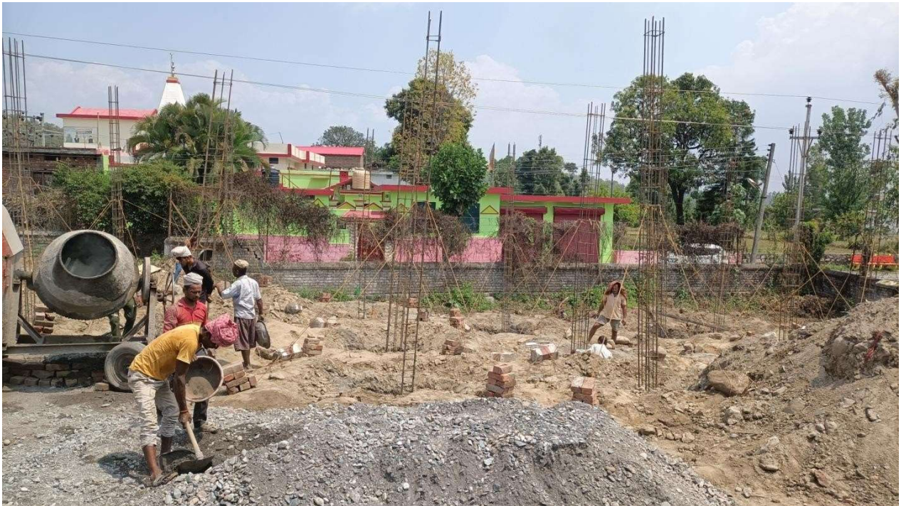
Foundation laying as per blue print
