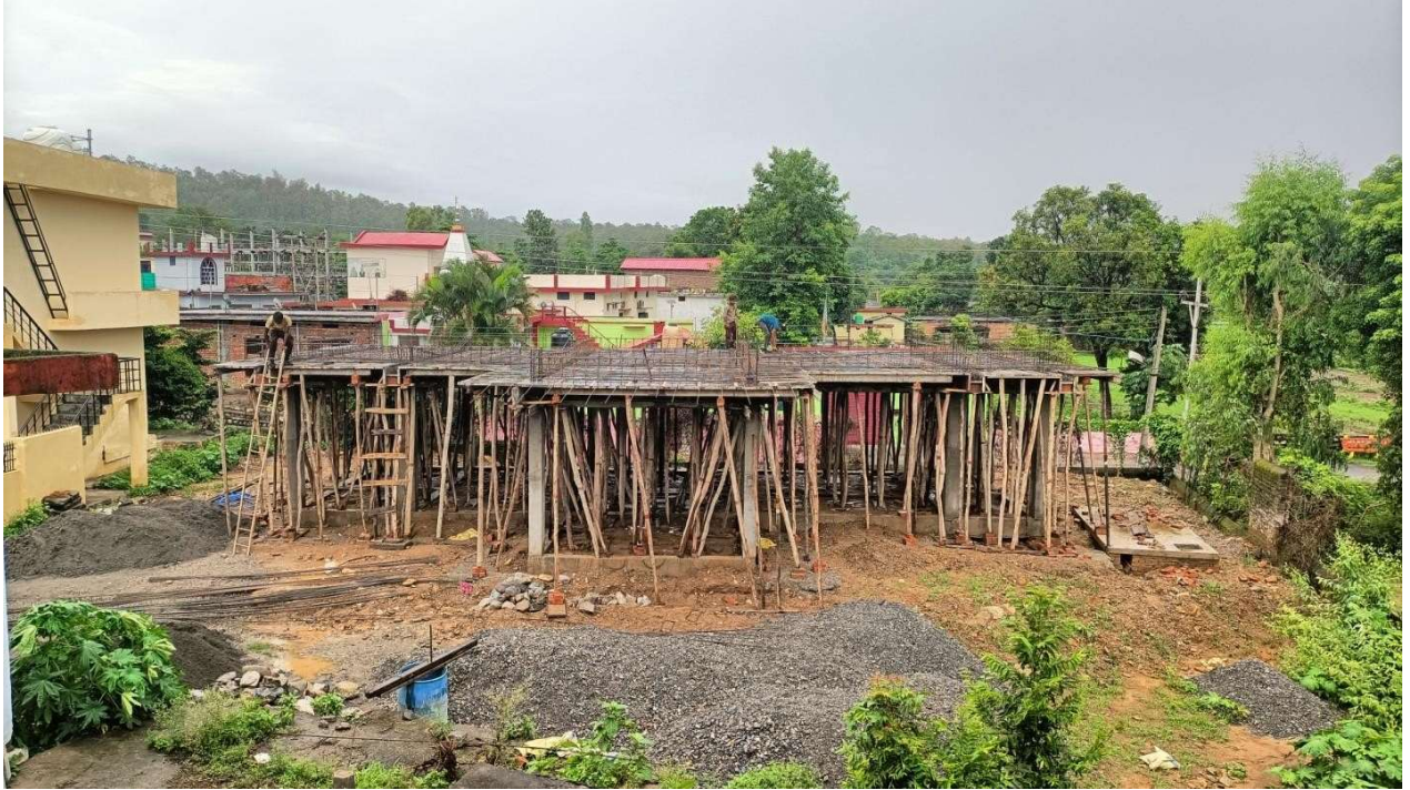
Setting for roof slab concreting of new office.
