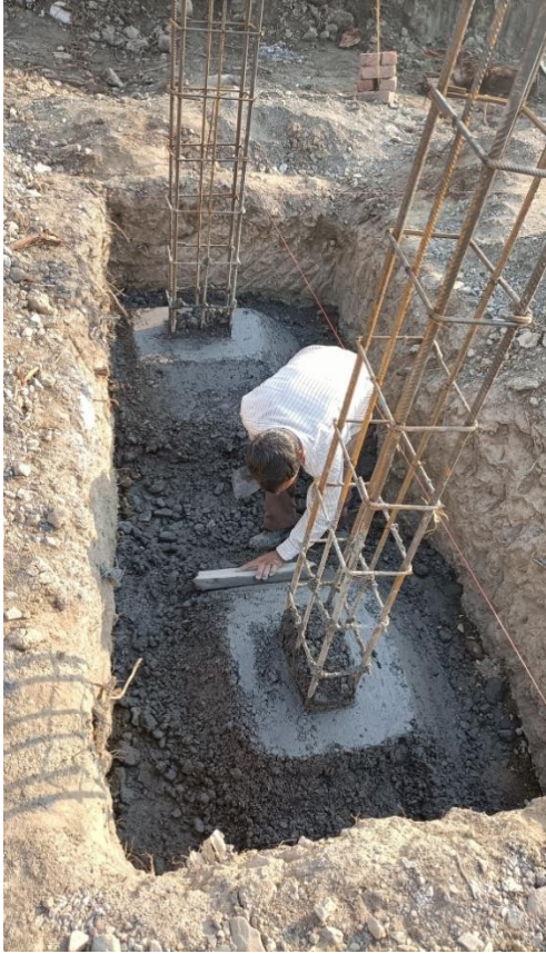
Pillar foundation Concreting.
