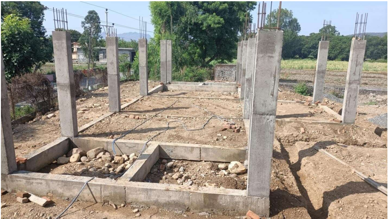
Foundation structure raised as per blue print.
