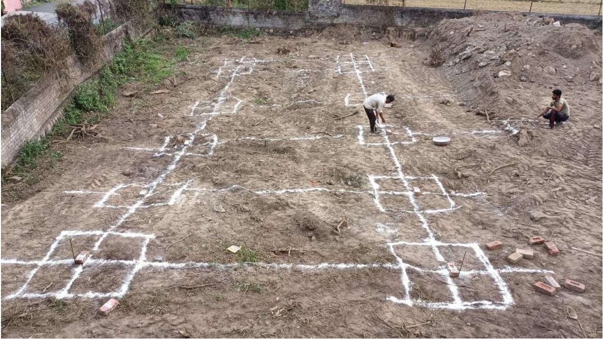
Marking for the foundation digging
