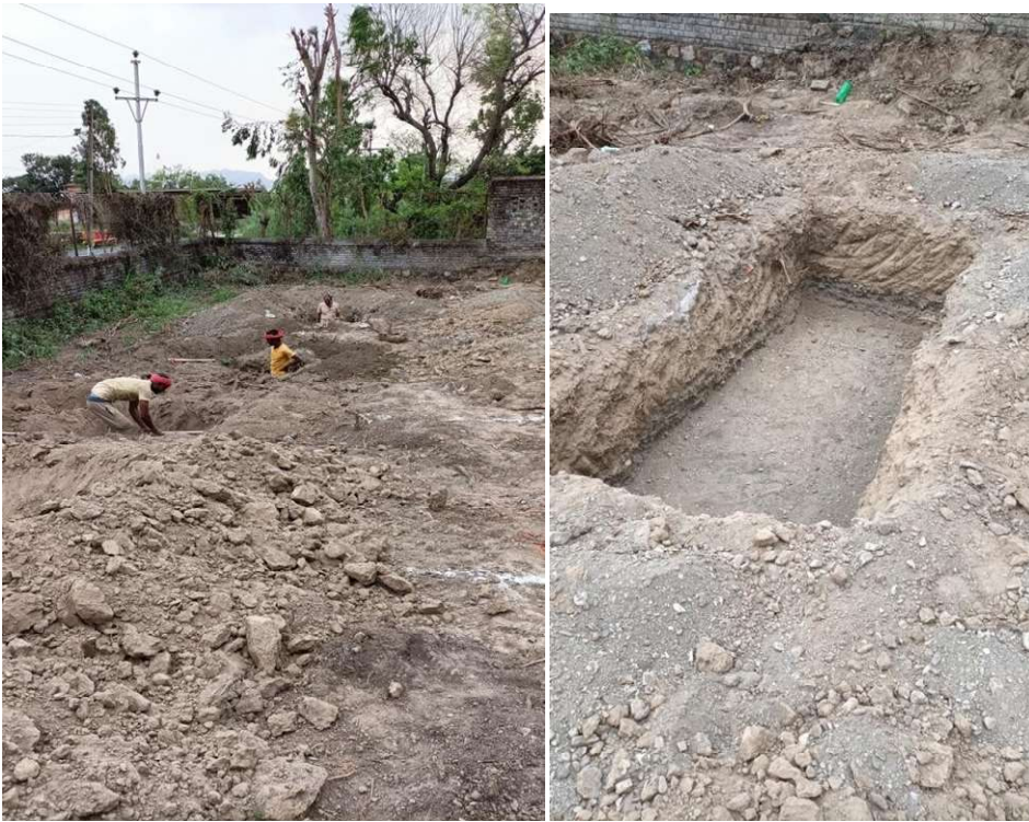
Digging foundation as per blue print
